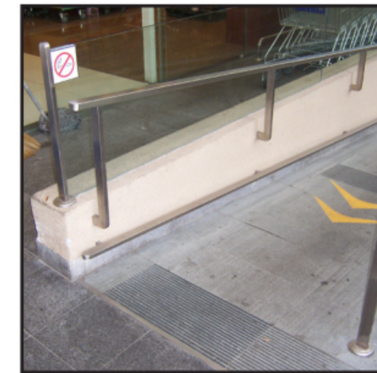
Tactile warning strip & clear indication of direction
